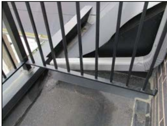
Modified bitumen membrane
