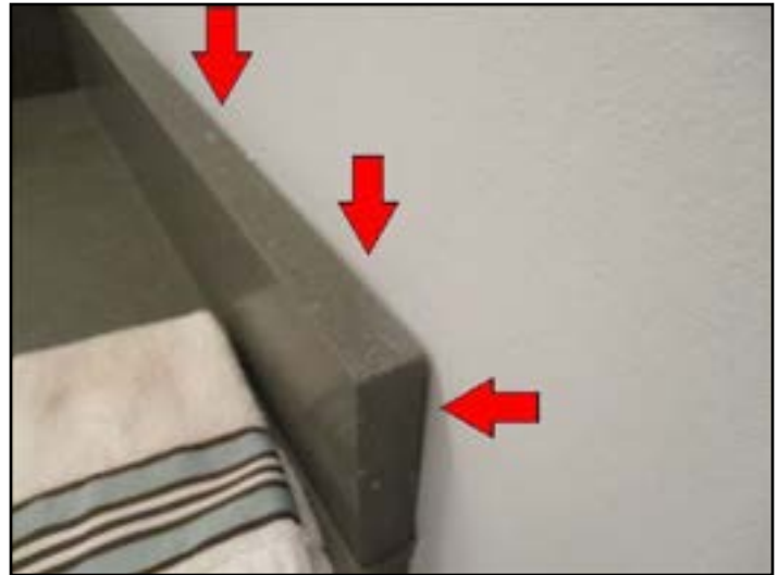
Example - missing sealant
