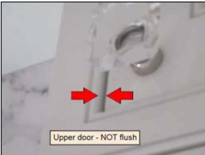
11.3 Cabinet doors or drawer faces are warped
