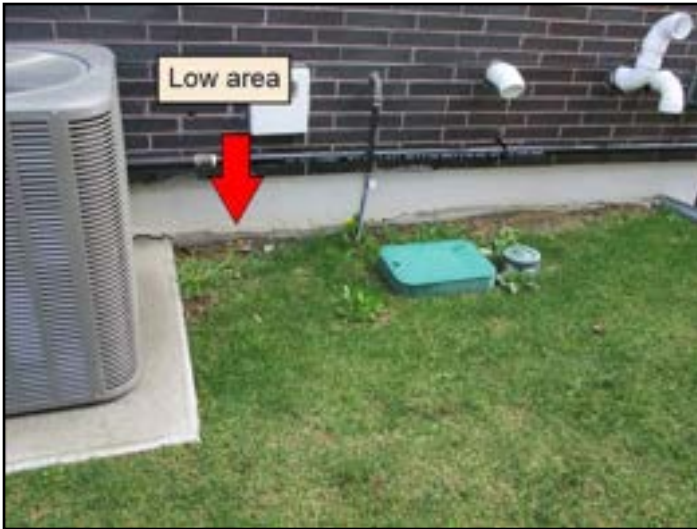
Improper slope or drainage
