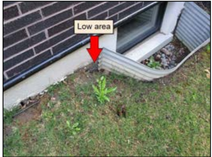
Improper slope or drainage
