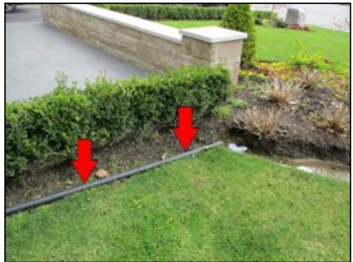
Discharge pipe problems
