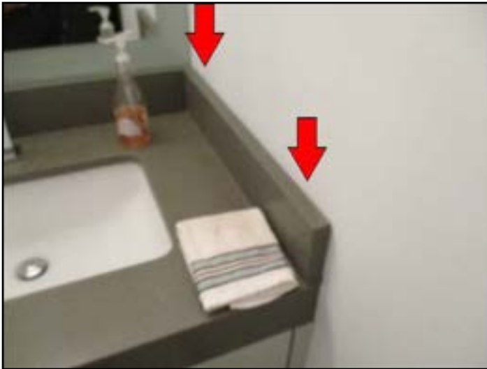
Example - missing sealant
