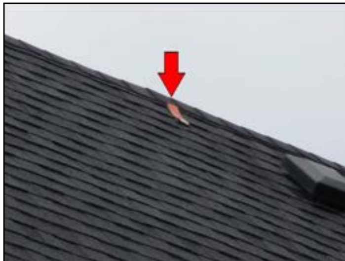
5.16 Temporary safety straps left on roof
