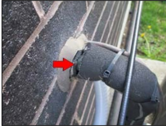
Insulation - missing
