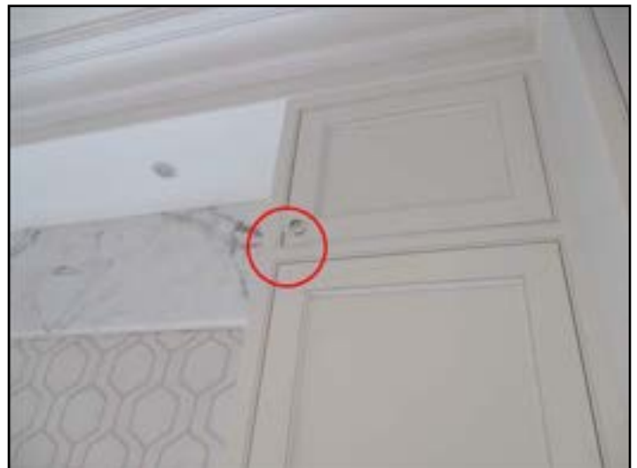
11.3 Cabinet doors or drawer faces are warped
