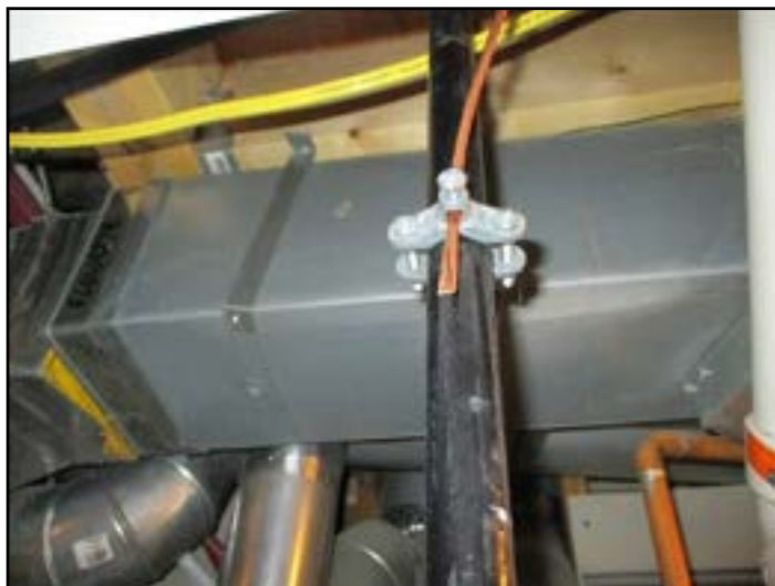
Bonding (for Gas Piping) present
