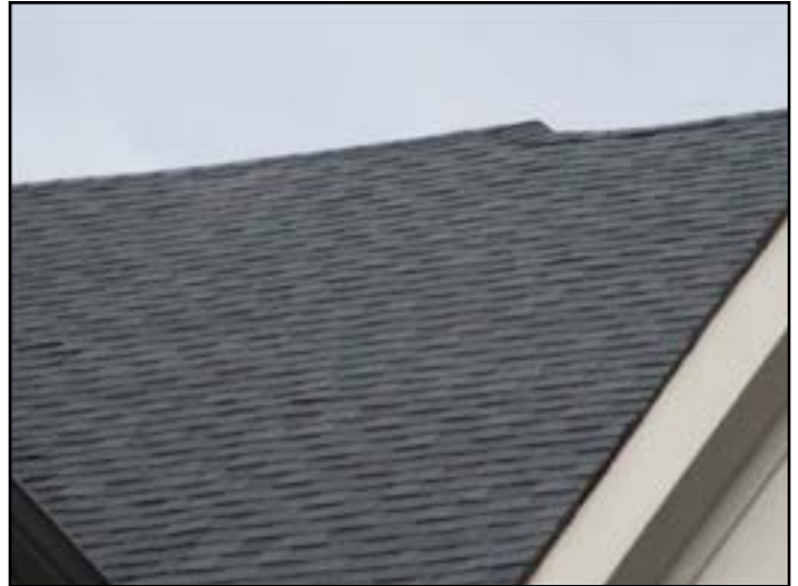
Asphalt shingles
