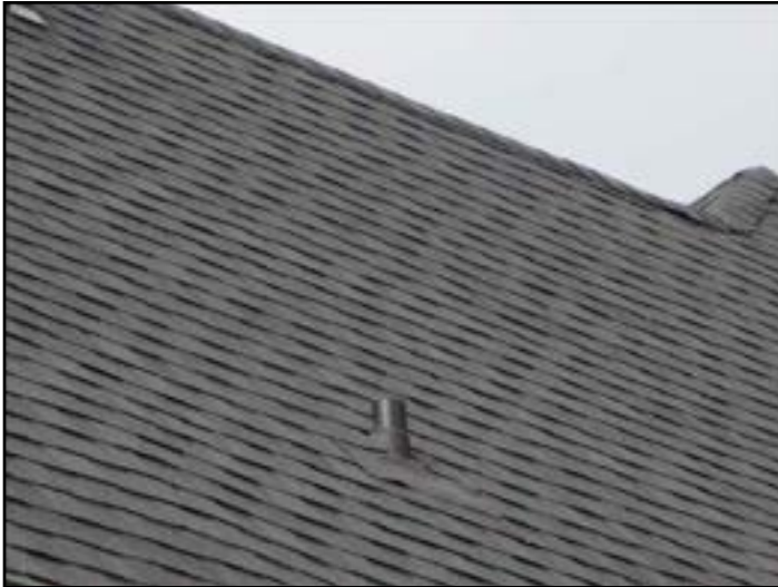
Asphalt shingles
