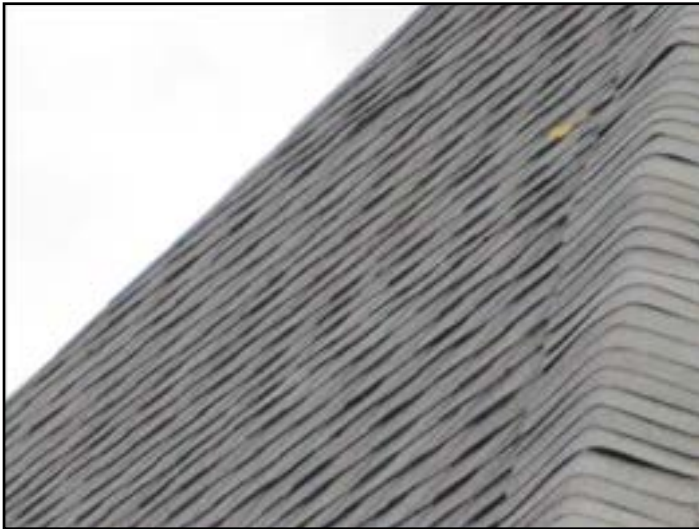
Asphalt shingles
