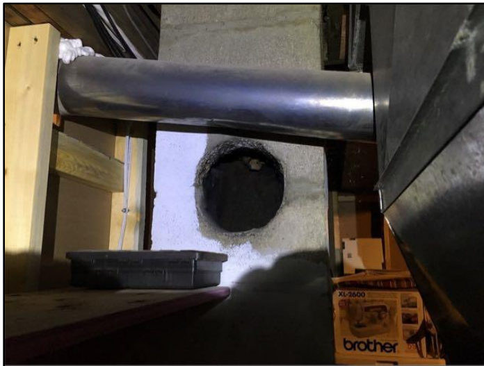
27. Abandoned openings for flue connections
