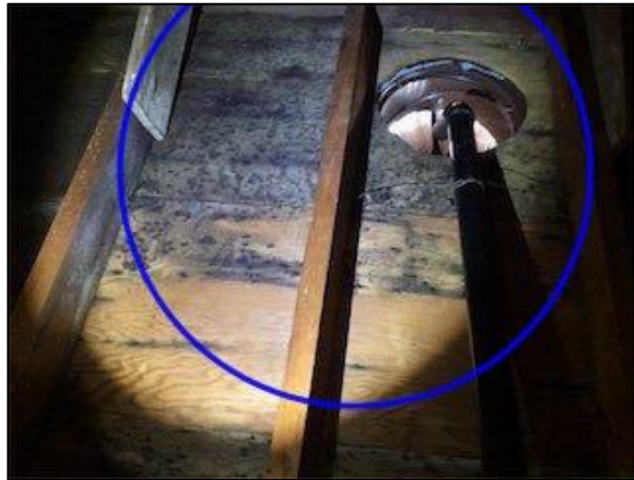
21. Attic staining on roof sheathing...
