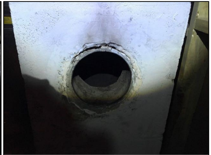
28. Abandoned openings for flue connections
