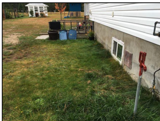
15. Improper slope or drainage
