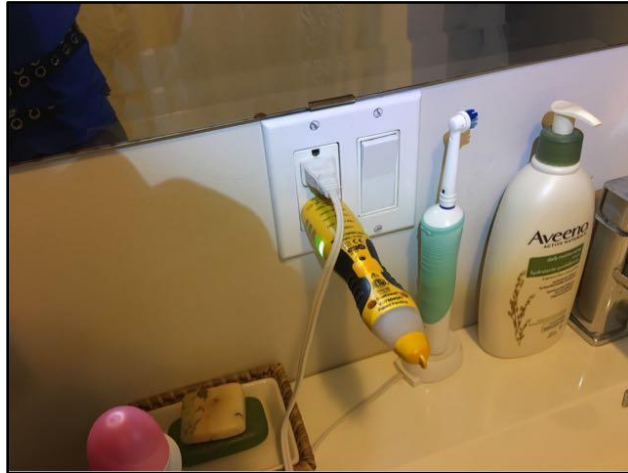
25. GFCI/GFI needed (Ground Fault Circuit...
