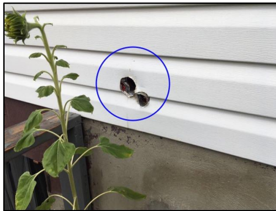
2. Seal all penetrations on exterior walls
