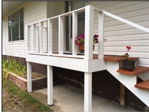
12. Openings between spindles (balusters) too...
