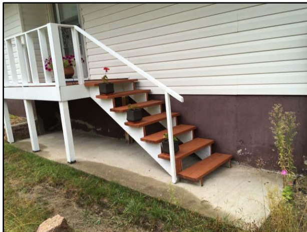
13. Spindles (balusters) missing
