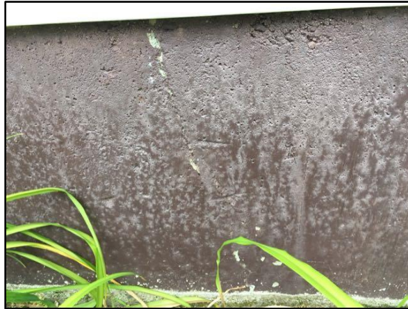
19. Typical minor cracks
