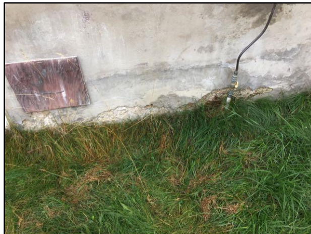
20. Parging damaged or missing
