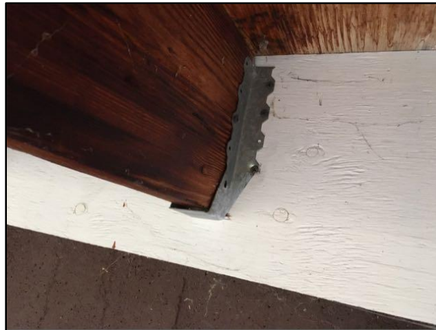
8. Improper fasteners on hangers
