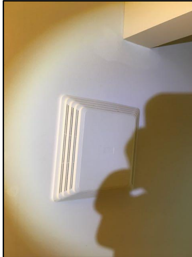
39. Inadequate air movement
