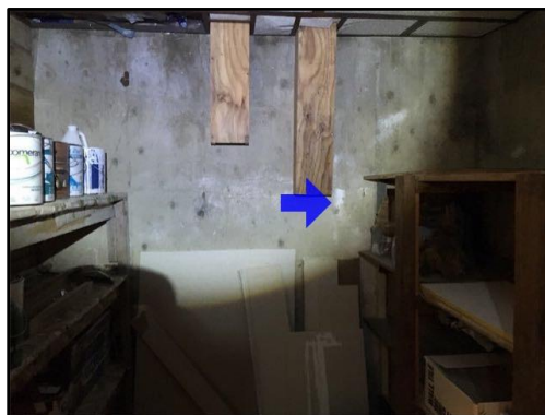
40. Efflorescence
