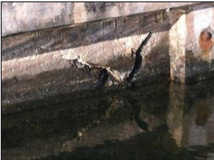
Spalled Concrete
