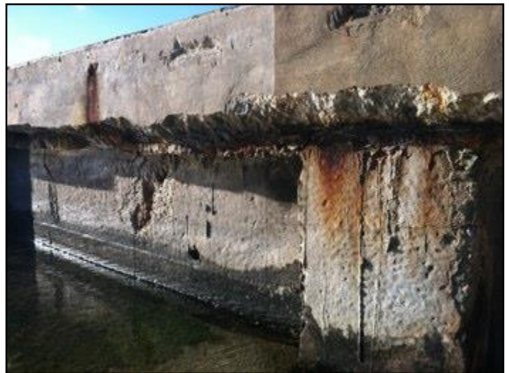
Spalled Concrete
