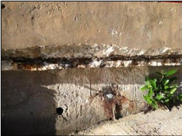
Spalled Concrete
