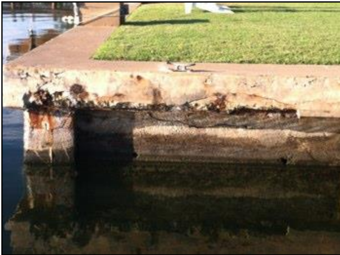
Spalled Concrete
