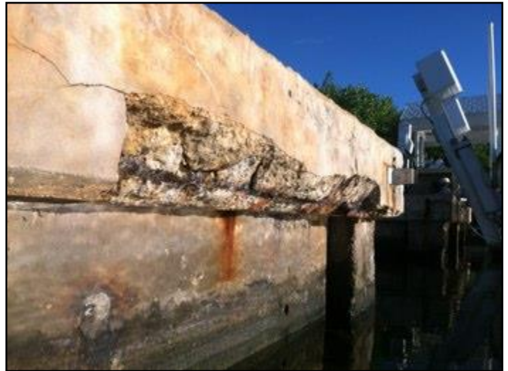
Spalled Concrete
