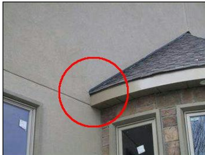
2. No kickout flashing
