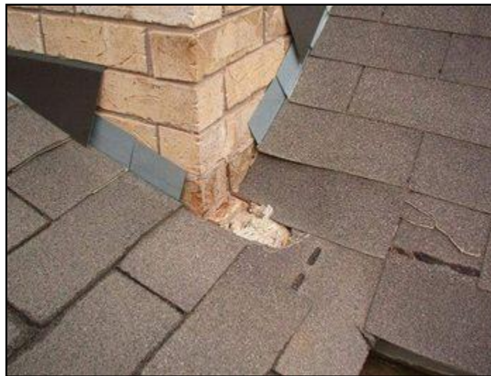
1. Missing top, bottom, side flashings
