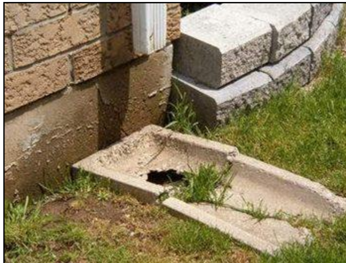
3. Downspouts end too close to building
