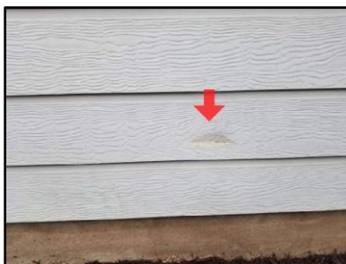
20. Mechanical damage
