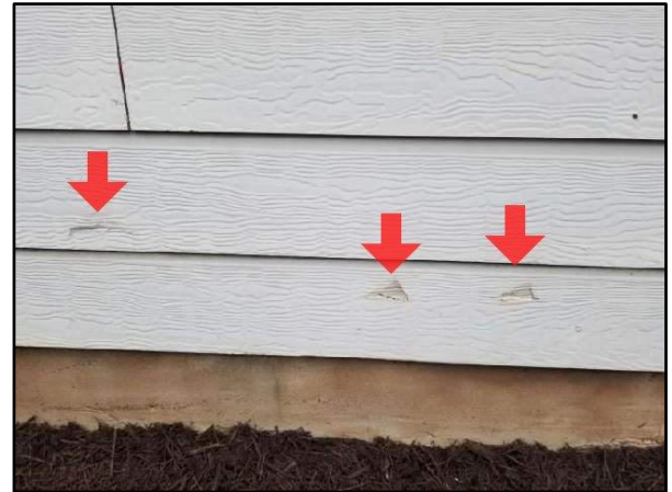
7. Mechanical damage
