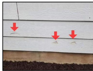
21. Mechanical damage
