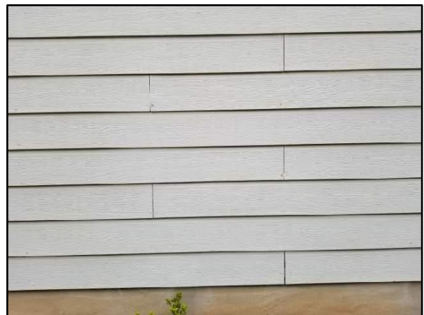
19. Siding runs right to horizontal flashings—a...
