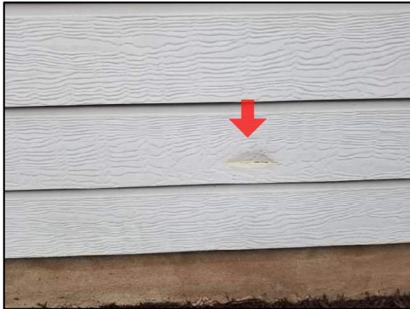
6. Mechanical damage
