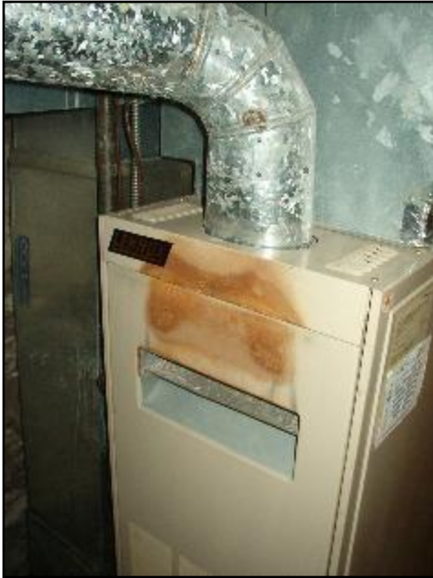
Draft hood spillage or backdraft
