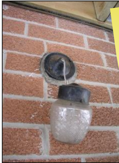
Light fixture is not well secured
