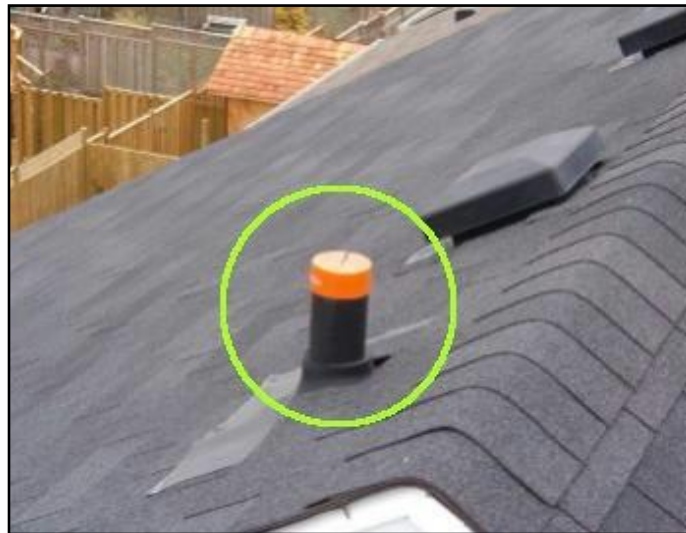
Plumbing stack is capped
