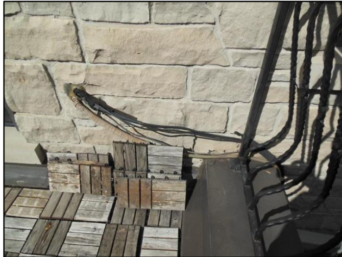
27. Insulation - missing
