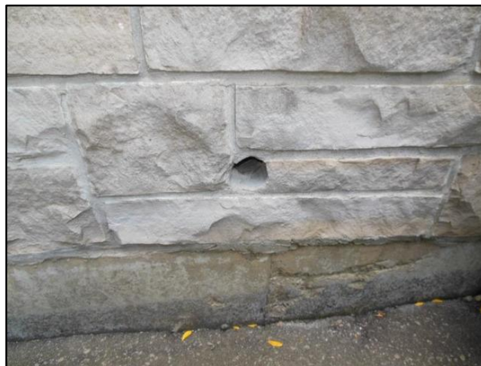
9. Mechanical damage
