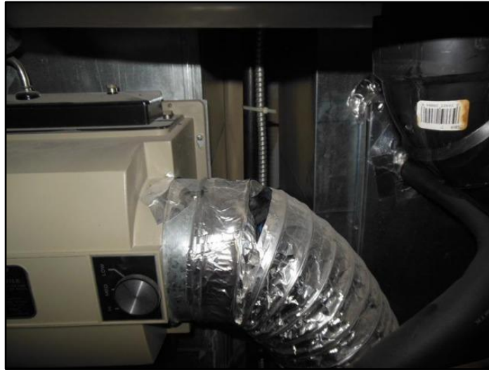
24. Ductwork damage
