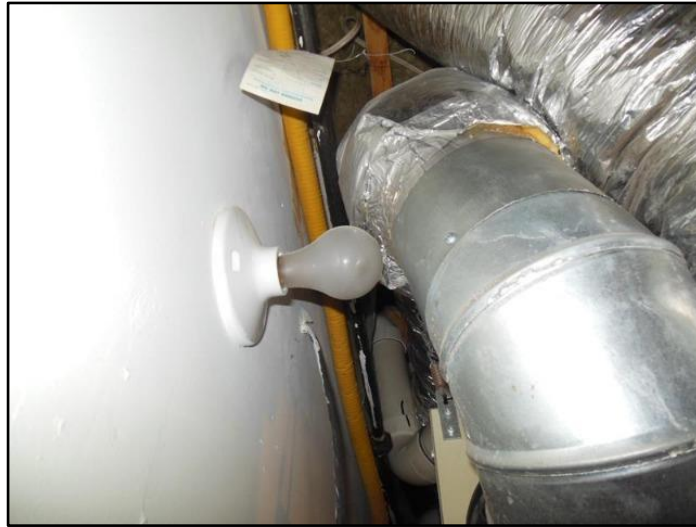
21. Exposed to mechanical damage (No cage or...
