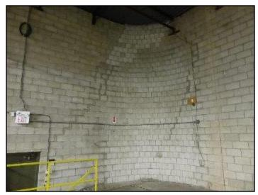
12. Minor settlement crack at southeast warehouse
