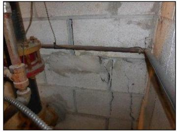
**11.** *Minor settlement crack in main electrcal room*
