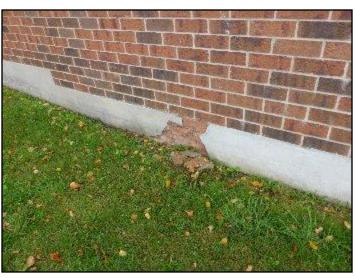
16. Spalled cement parging
