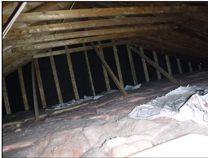
Glass fiber - example - lower attic
