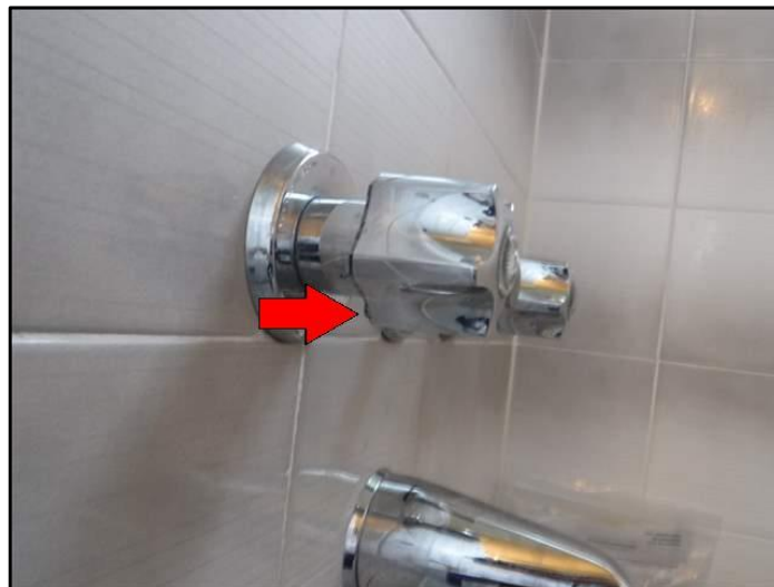
Leak - hot water
