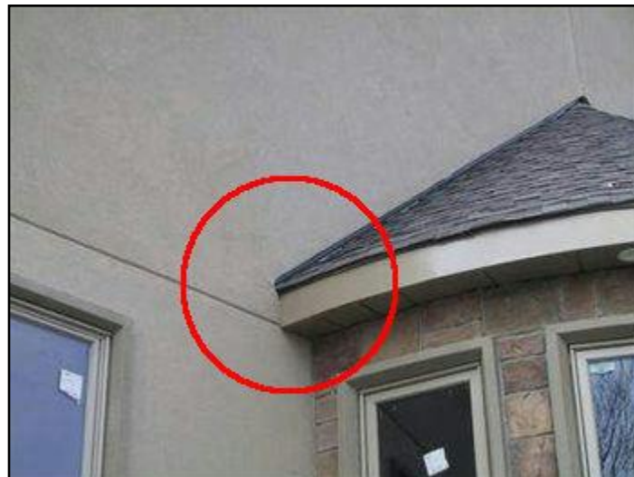
2. No kickout flashing
