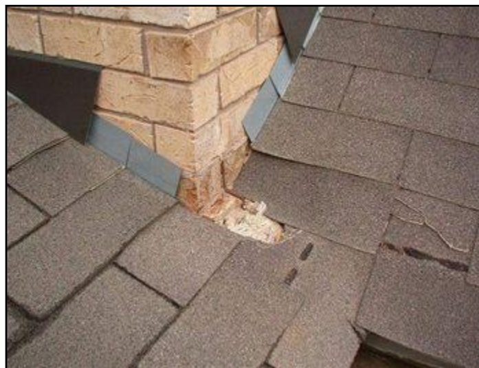
1. Missing top, bottom, side flashings
