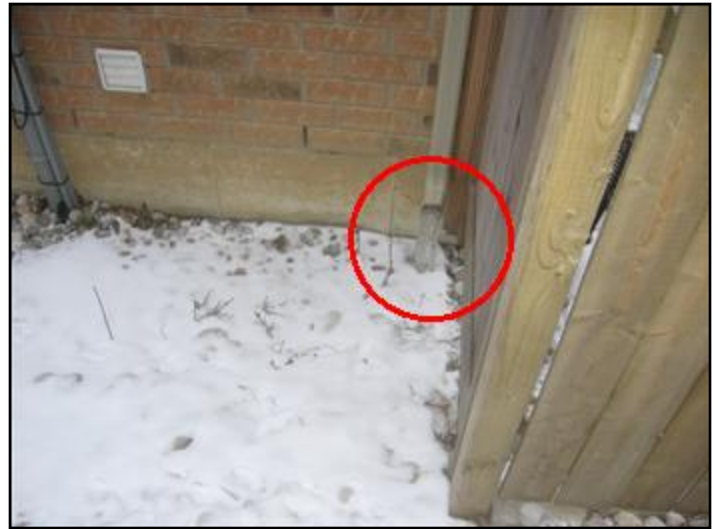
at NE corner
