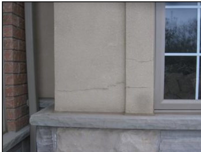
at west wall
