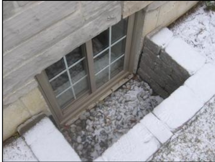
deep window well
