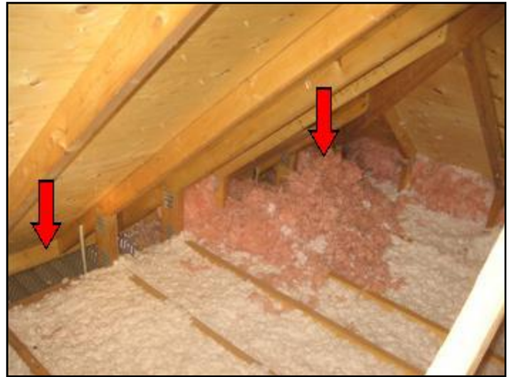
insulation has been moved to make a nest
