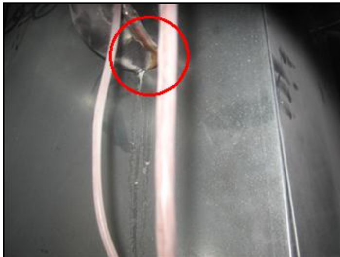
seal to prevent cold air loss
