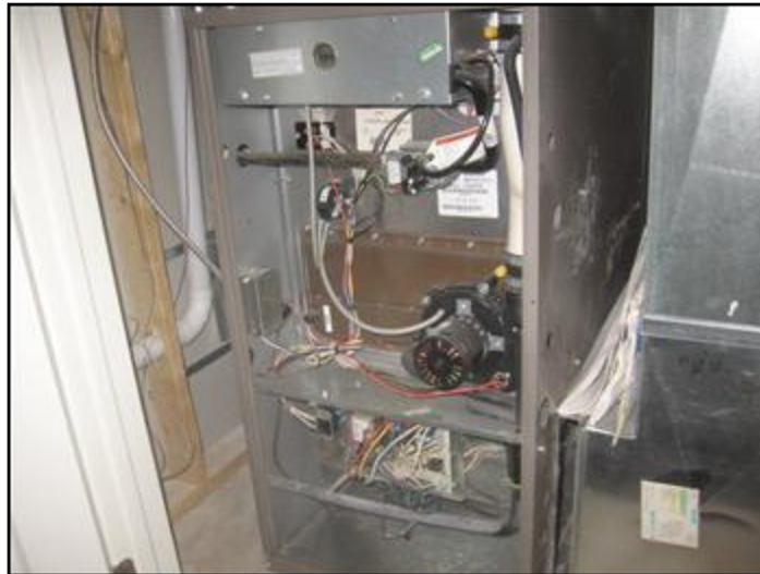
high efficiency gas furnace
