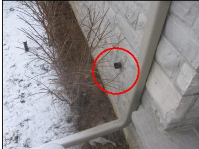
provide extension on discharge pipe
